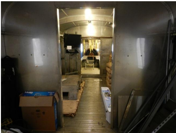
"A" Power Car - Looking into the engine compartment. The Flying Yankee Restoration Group is looking into a new engine, replacing the old Winton "A" Diesel Electric Engine which was removed a long time ago.
