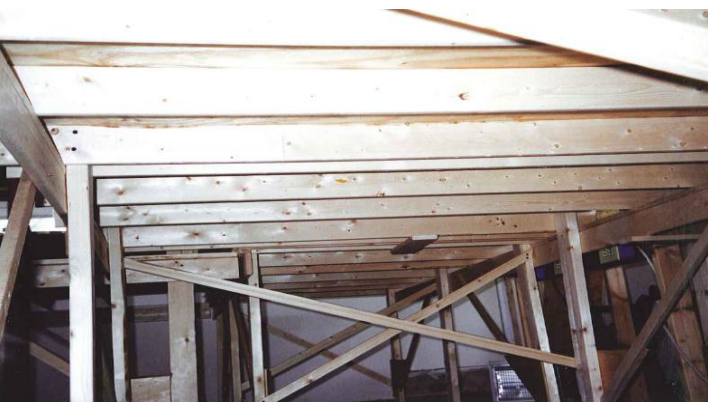
Under the layout after a few L-Girders are built and together
