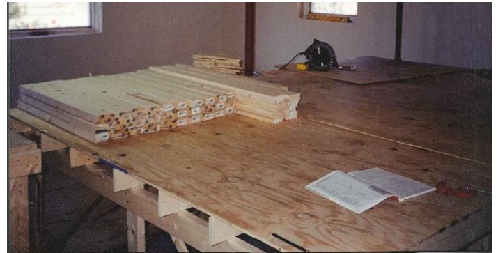
Lumber for the L-Girders
