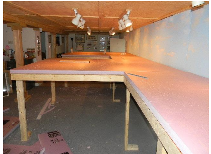
Pink foam attached and the walls painted blue.
