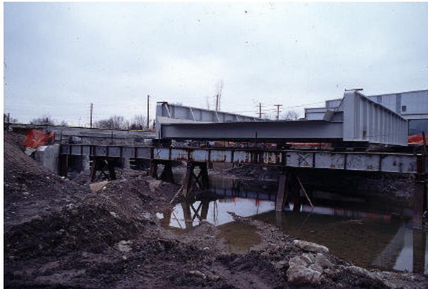
Photographing the new bridge from the creek bed shows the new bridge completed. The last of the horizontal I beams was installed closest to the old bridge. A layer of track blast was placed on the deck of the new steel bridge. By the middle of December, the new bridge was less than two weeks away from being installed.
