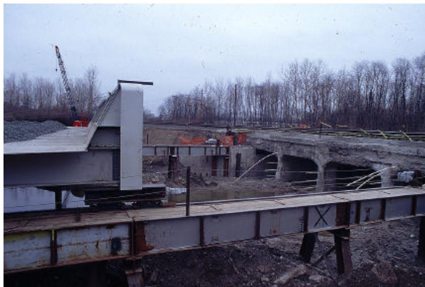
Looking north at the bridge project, here is a good view of the PVC pipe on the old bridge. Workers drilled deep holes in the deck and supports of the old concrete bridge, and then PVC pipe was inserted into the drilled holes. This will guide the dynamite in side the old bridge.
