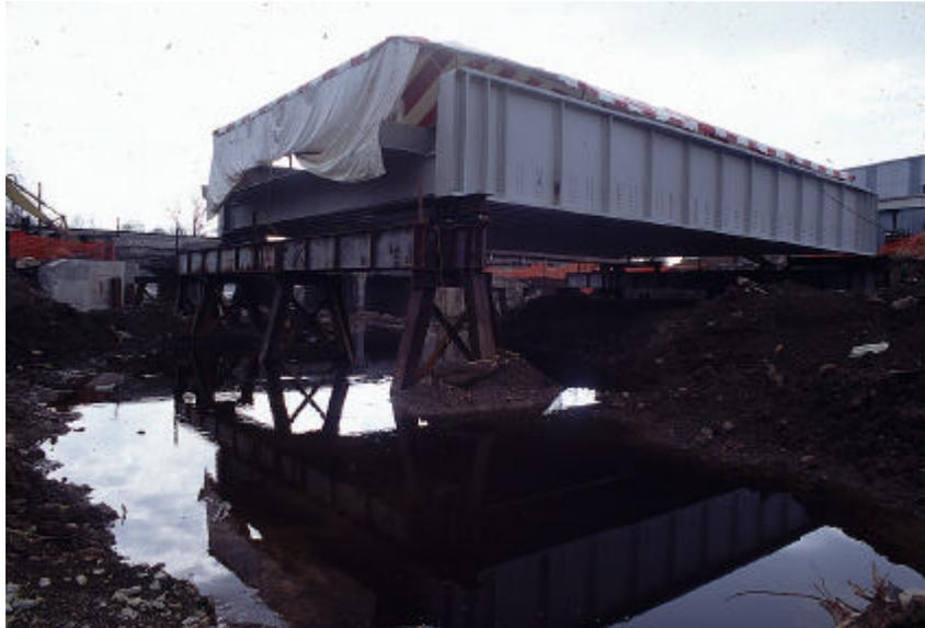
In this view we are looking east from the creek bed. This is a good view on how the bridge was supported above the stream during construction. There were no problems with high water during this project, they were lucky, it was a dry late fall and early winter. Photo by Bradley McClelland
