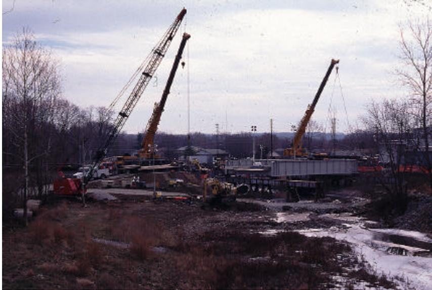
In this view we can see that the old concrete bridge was removed. Two large yellow cranes spotted on the tracks will lift the new steel bridge to its final home. The one crane on the south bank has its cables connected to the new bridge. In the creek bed where the old bridge used to be, a backhoe with air hammers blast away at the remaining concrete supports. Too the far left, a stack of new track is waiting to be placed on the steel bridge.
