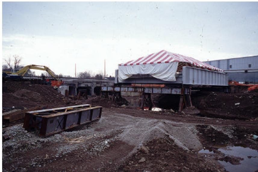
This is a good view of how the through girder bridge was built above the stream bed. The double steel I beam on the ground to the left will be added to the rest of horizontal I beams, The new bridge will roll on top of horizontal I beam to the tracks. We are looking south in the picture. Photo by Bradley McClelland
