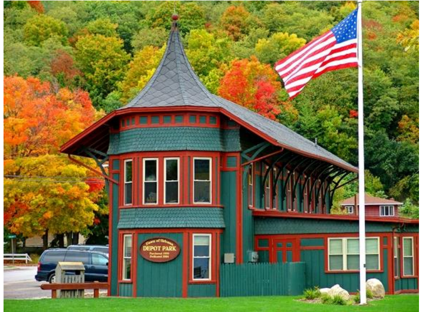
Bath & Hammondsport Railroad Passenger Depot, Hammondsport, NY.
