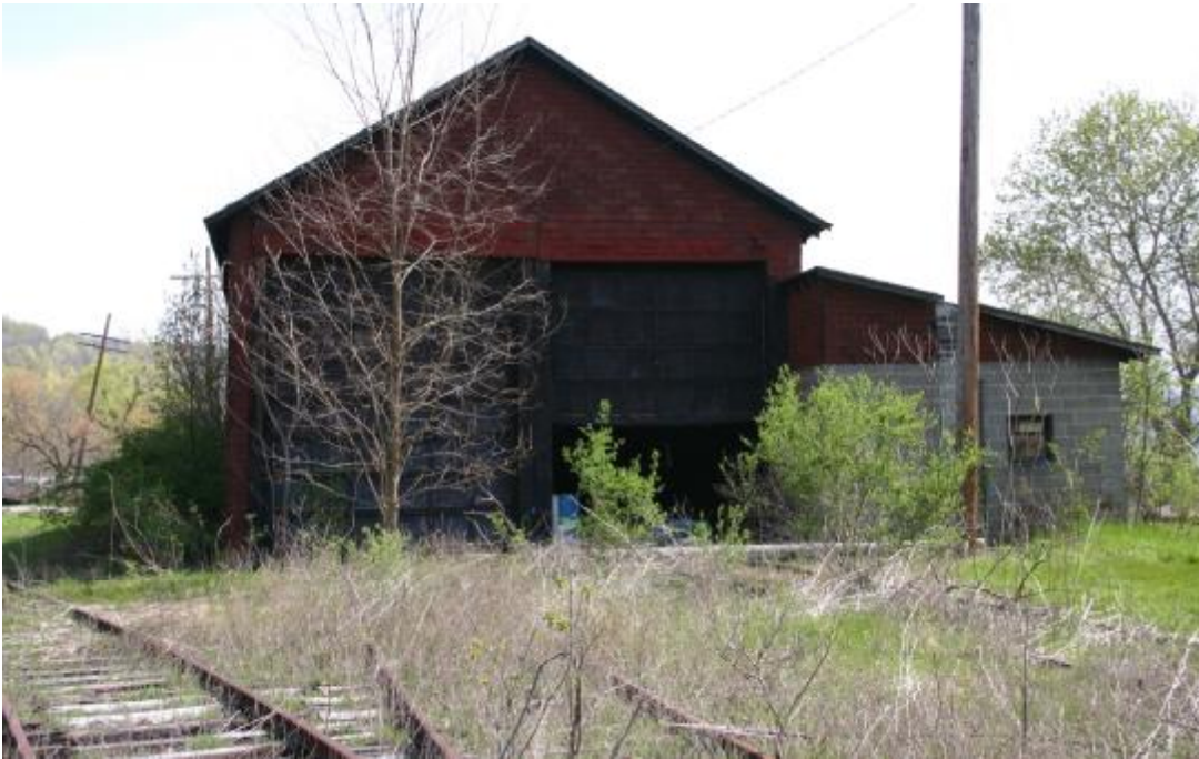
The Bath and Hammondsport Railroad Engine House, May 2006. View is looking north at the south end of the Engine House.
