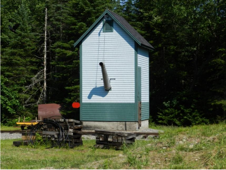
Enclosed water tank, stacks of rail ties in front and rail work cart in the rear.
