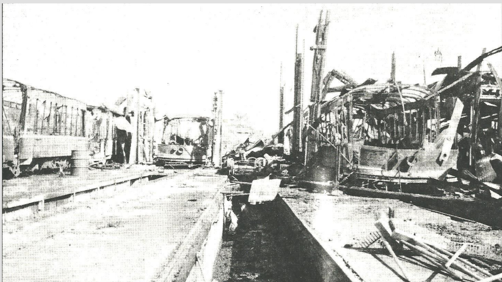
(This was once the Phoenix car barn. Note how the intense heat of flames melted and twisted track, cars and girders. Car 505 at the right.)
