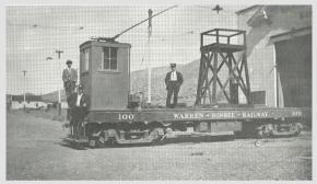
tially from 101 to 107. They were 42 feet in length with seating for 40 and standing room for 75 and were equipped with 40 hp motors necessary for the steep grades encountered. The line could be technically an interurban since it served different urban centers and had large MU-capable cars; however, it operated more like a streetcar line with little private right of way, and mostly street-running.
