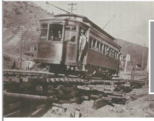
Car 103 crossing a washout over temporary trackage. to be built on the narrow Main Street, the car line did run up Main St. in Bisbee in a steep, twisting route. In 1909, the line was extended past downtown Bisbee up Tombstone Canyon past Castle Rock. The electric line eventually reached its maximum length of 12 miles, using 60 lb. rail and 80 lb rail on the steeper grades. The carbarn was located
